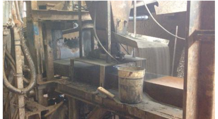
SHOWER of MATERIAL OVER BRICK SURFACE
