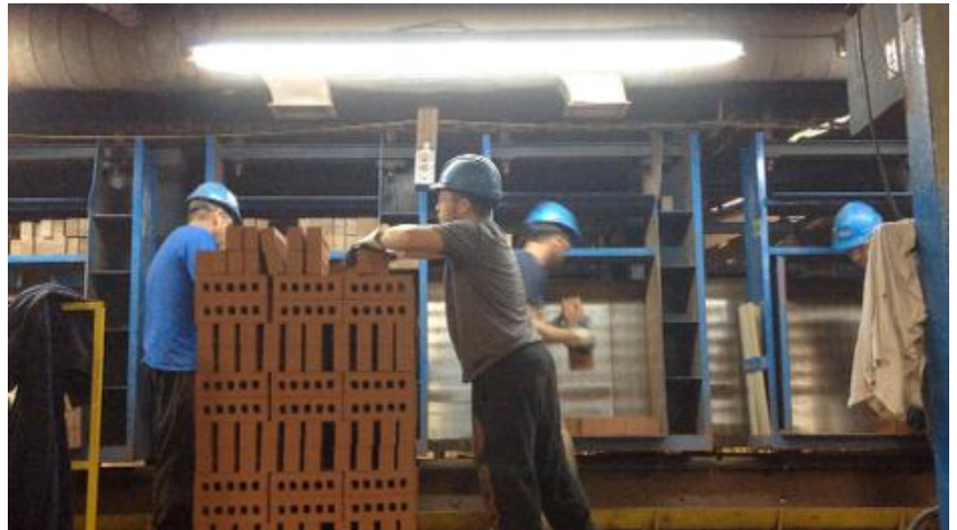
A VERY INTERESTING QUALITY CONTROL CHECK: BRICKS TAPPED AGAINST EACH OTHER!!!
