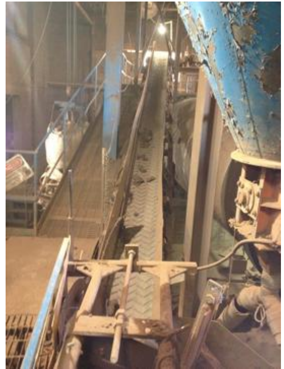
CLAY BEING CONVEYED to MIXER
